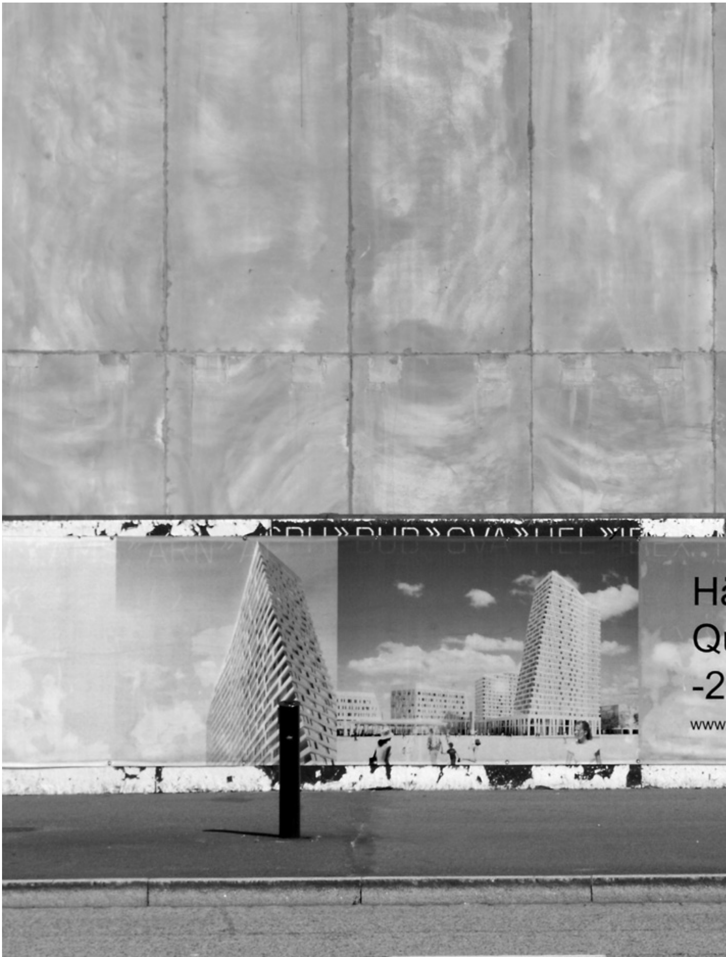
The hoarding on the site indicates that there is a certain amount of simulation going on. The text reads: "Quality Hotel View, Point Hyllie, opening here 2015."
